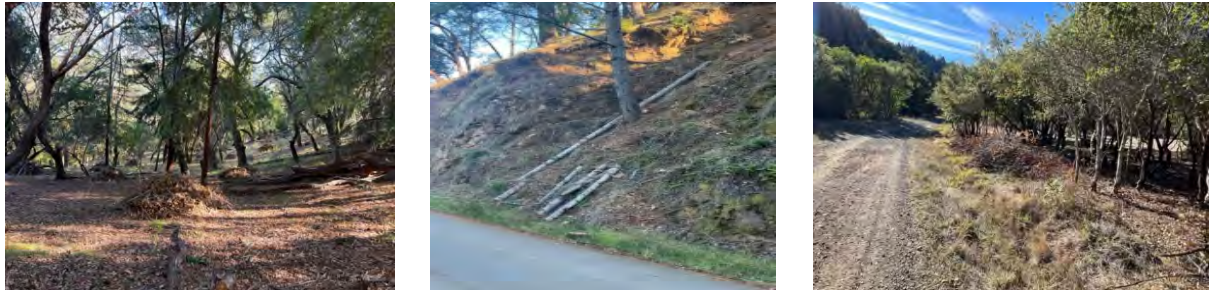
Figure 1-8. Examples of Fuel Treatment, Fuel Breaks, and Roadway Work
